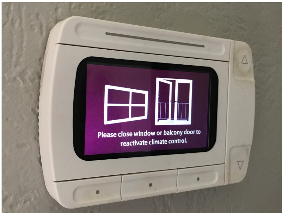
Figure 18. Auto shut-off control for air-conditioning based on natural ventilation
