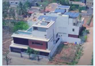
Residence of Mr. Selvarasu
