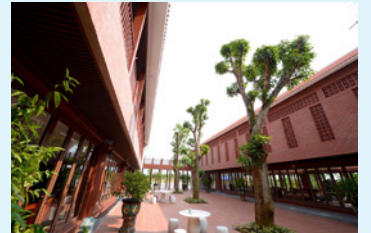
Song Duong River Surface Water Treatment Plant
