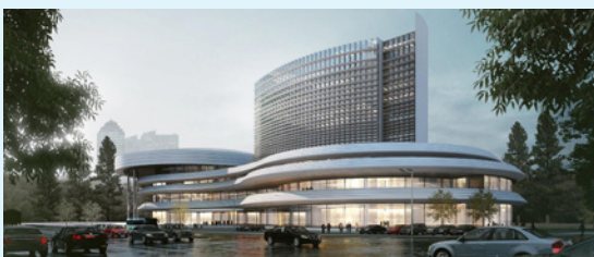
Bac Ninh Exhibition Center of Urban Development and Architecture
