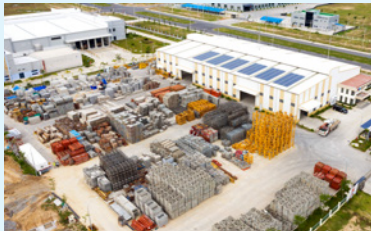
Ricons Mechanical Processing Plant-Phase 1
