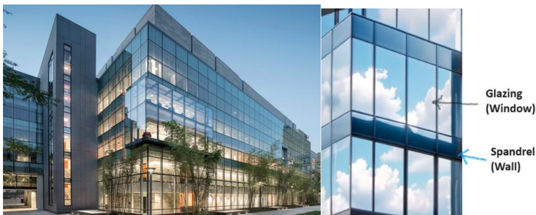
Figure 3. Window to Wall Ratio of Building with Curtain Wall Glass 2
